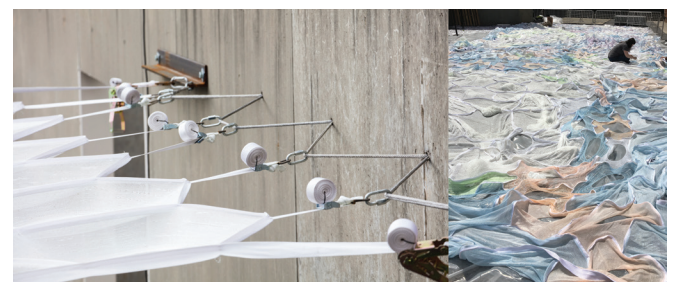
21 Perimeter edge details (left) and unfolding and preparing the canopy for installation; solar active yarns revealing their colors in the presence of the sun (right).
