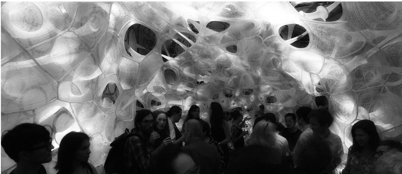
10 Interior shot on opening night. The entire structure is pulled into tension, cone by cone, until the bottom forms a taught elliptical tension ring
